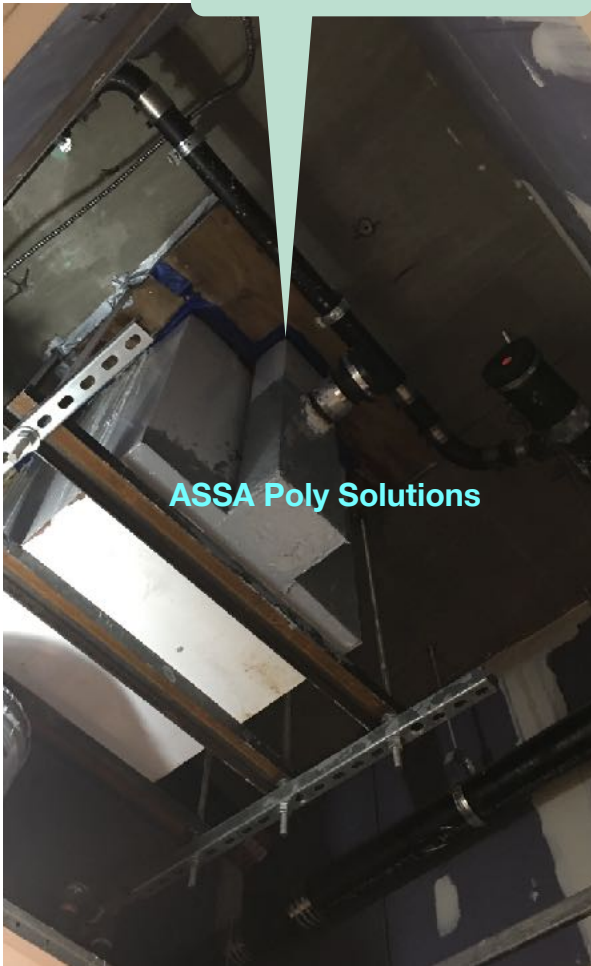
Exterior outlet pipe wrap repair
